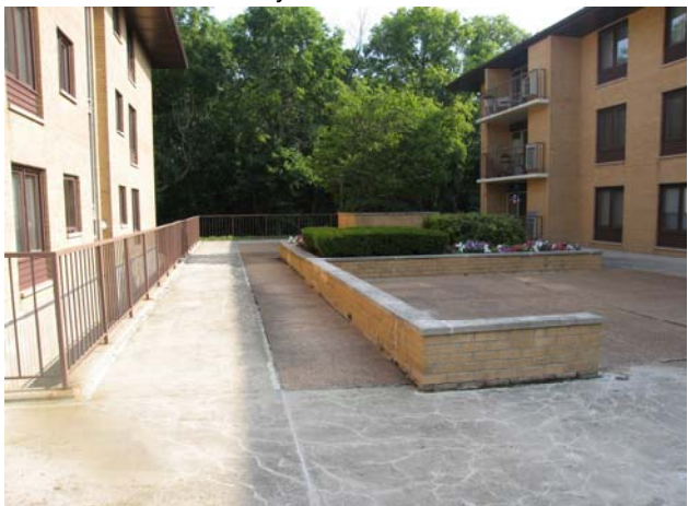
View of Courtyard Prior to Renovation
