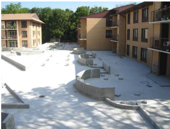
Construction Photo of Renovation
