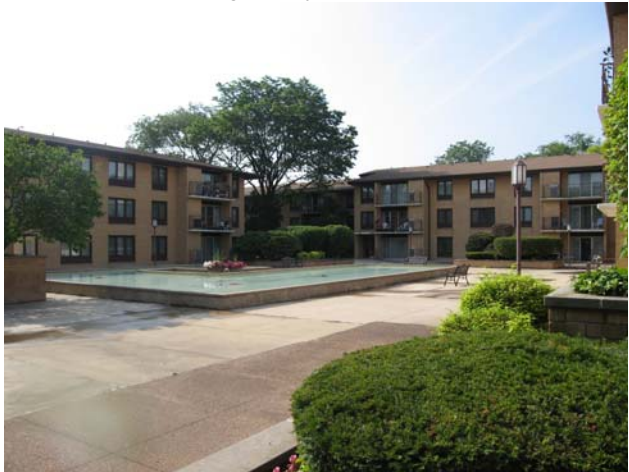
View of Courtyard Prior to Renovation
