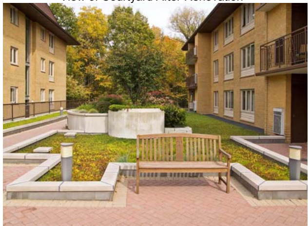
View of Courtyard After Renovation
