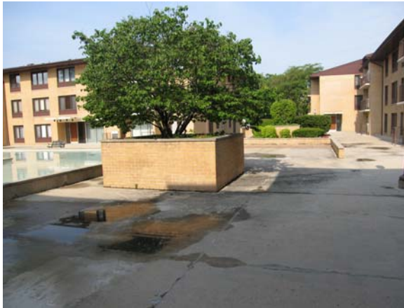
Courtyard Prior to Renovation
