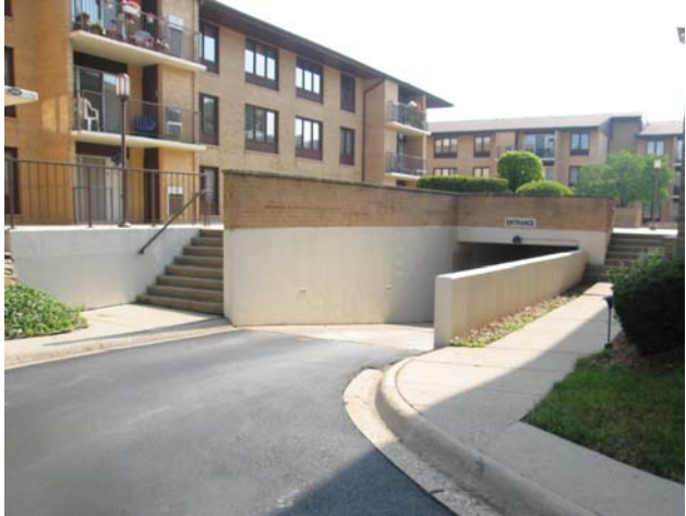
View of Garage Entry Prior to Renovation
