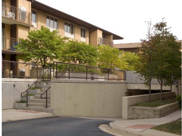
View of Garage Entry After Renovation
