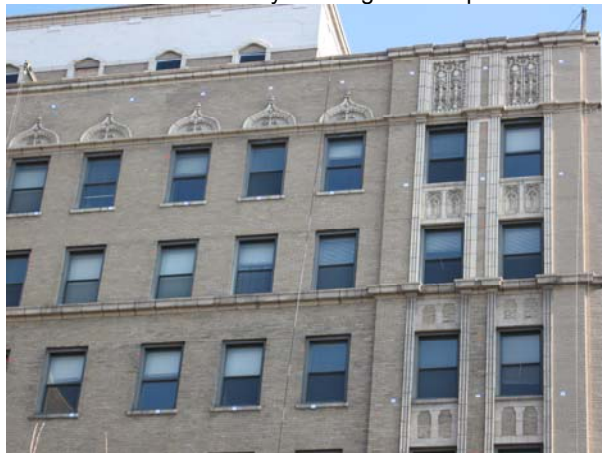
Close-up View of Terra Cotta and Brick Masonry
