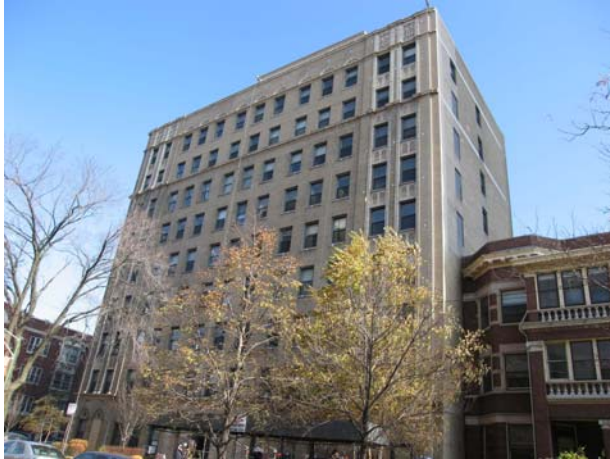
View of the Nine-Story Building after Repair Work
