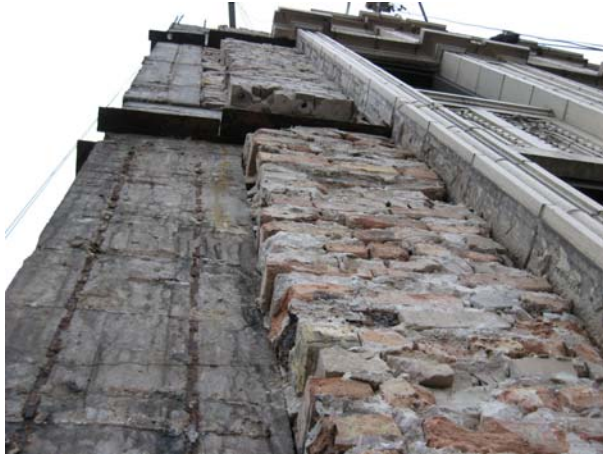
Demolition: Building Corner
