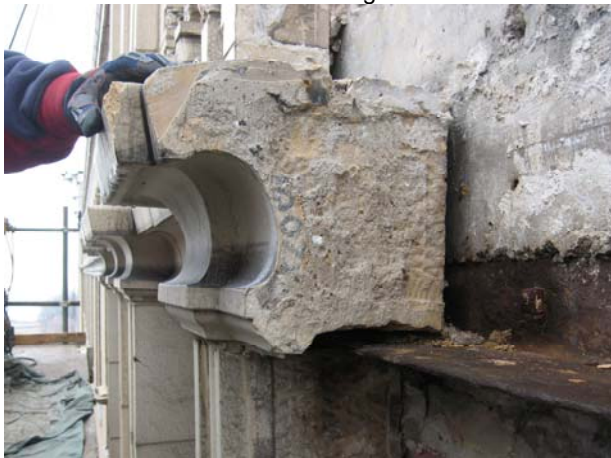
Salvaged Terra Cotta Repairs
