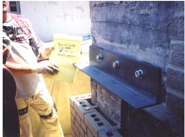
Installation of Replacement Shelf Angles
