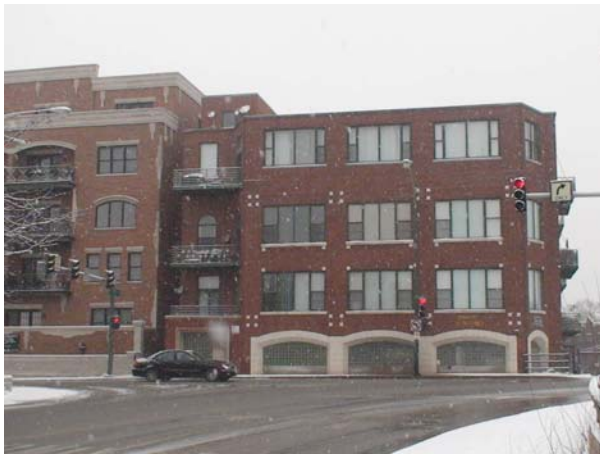
River Park at Diversey Condominium, Chicago, IL Loft Conversion Monolithic Brick Masonry Building
