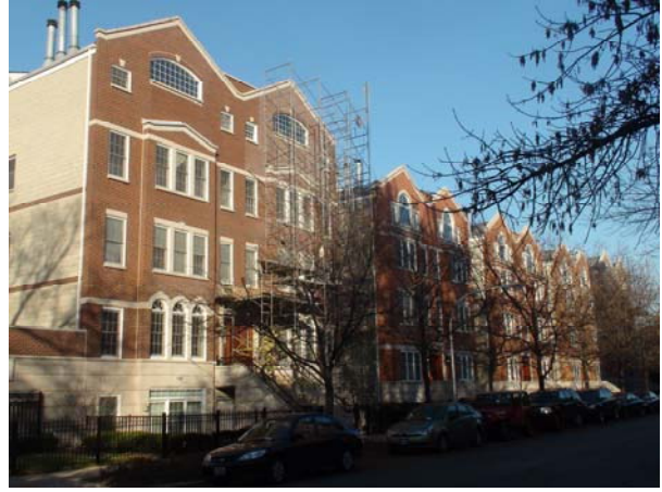
1300 - 1322 West Fletcher Condominium, Chicago, IL Five Brick w/ Concrete Block Backup Building Complex (1999)
