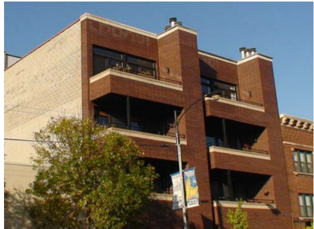
2308 West Chicago Condominium, Chicago, IL Brick w/ Concrete Block Backup Building (2002)
