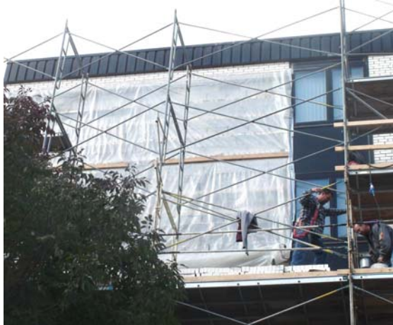
Prototype Wall Replacement in Progress
