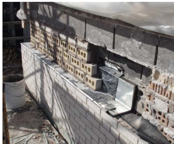
Shelf Angle Installation at Prototype Wall Assembly
