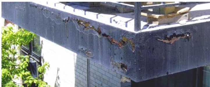
Close-up Photos of Typical Balcony Deterioration
