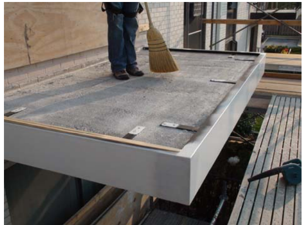
Installation of New Topping Slab and Matching Perimeter Steel
