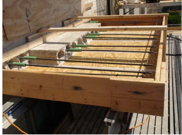
Replacement of Steel Reinforcement, prior to Casting Deck
