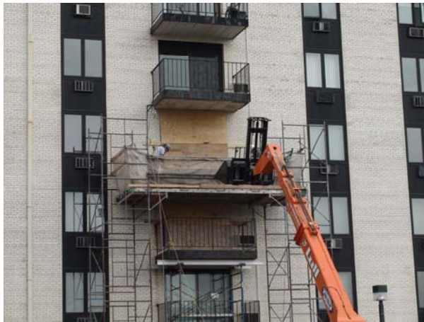
Pouring the Replacement Balcony Concrete Structural Deck
