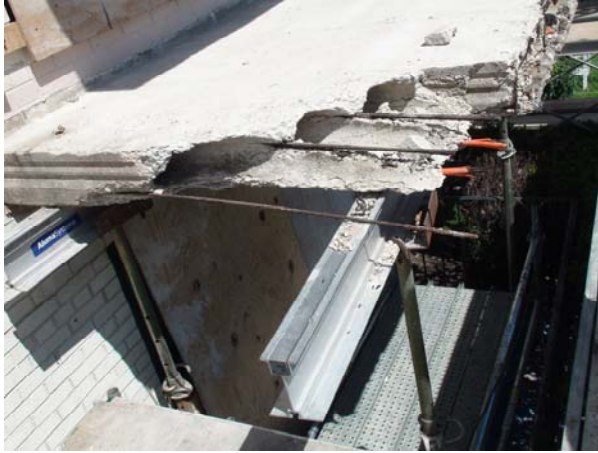
Partial Demolition of Existing Distressed Balcony
