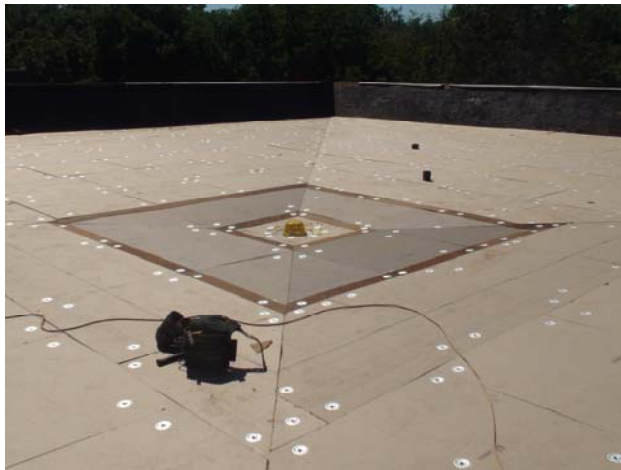
Installation of replacement R-20 Insulation
