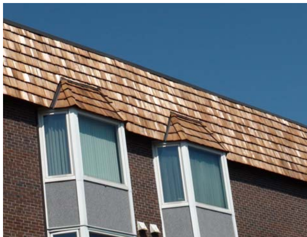
Detail of Cedar Shake Replacement Roof Assembly
