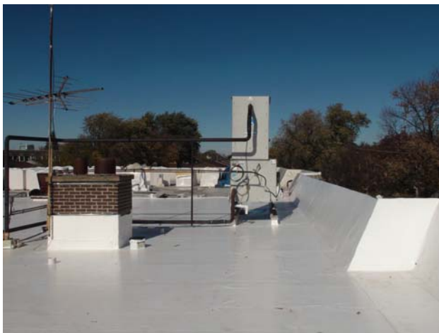
View of Completed Replacement Roof
