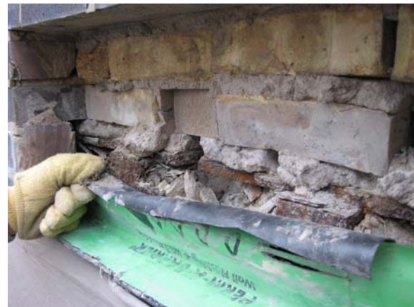
Flashing Set Into Inspection Opening, Prior to Rebuilding
