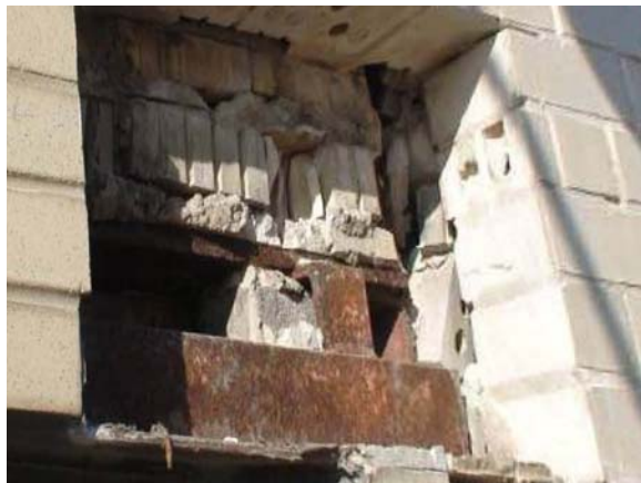
View of Typical Inspection Opening
