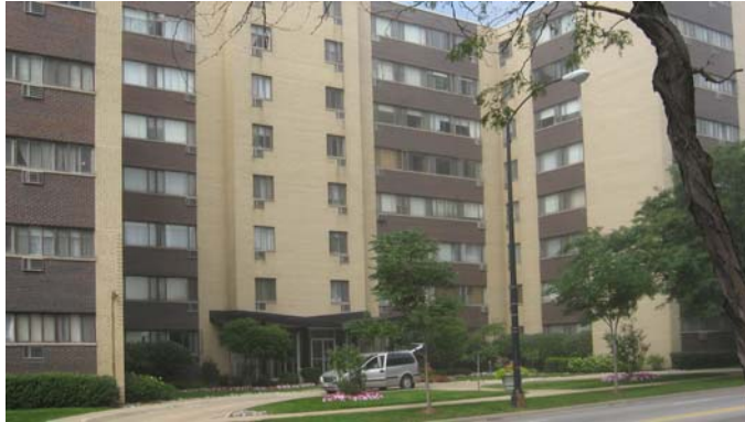
View of the 8-story, 126-unit Condominium Block
